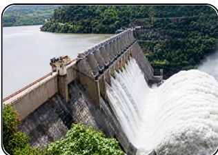
Bhakra Nangal Dam
